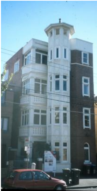
The Canterbury Flats, 236 Canterbury Road, St Kilda, 2002
